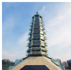
(c) Glazed Tower Wings of the New Nanjing Porcelain Tower
