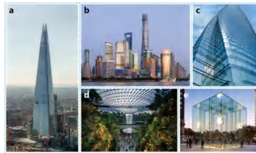
Figure 2 Typical Glass Curtain Wall Architectures[6]: (a) Shard, London; (b) Shanghai Central Business District; (c) Shanghai Tower; (d) Jewel Changi Airport, Singapore; (e) Apple Store on Fifth Avenue, New York
