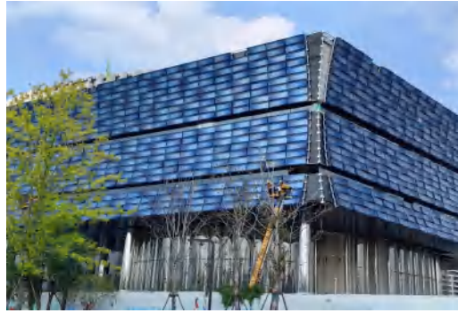
Figure 7 Outward-Tilted LIULI Composite Panel
