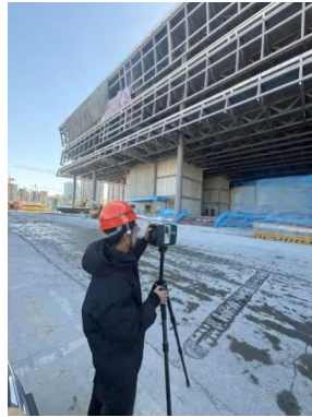
Figure 12 3D Laser Scanning
