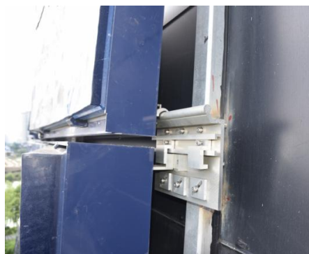
Figure 19 Panel Hoisting, Supporting, Alignment, and Locking
