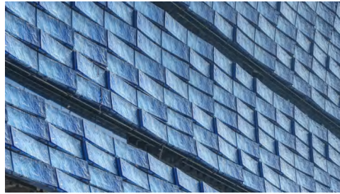
Figure 23 As-Built Appearance of the Large-Area LIULI Curtain Wall
