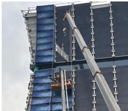
Figure 18 Dual-Machine Hoisting Using Truck Crane and Articulating Boom Lift
