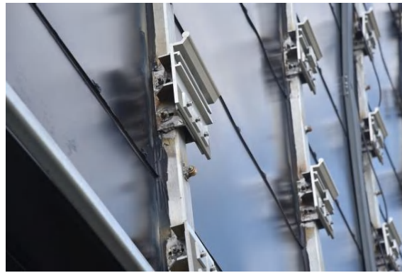
Figure 17 Precise Layout of "Bottom-Support and Top-Hook" Aluminum Alloy Brackets
