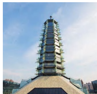
(c) Glazed Tower Wings of the New Nanjing Porcelain Tower
