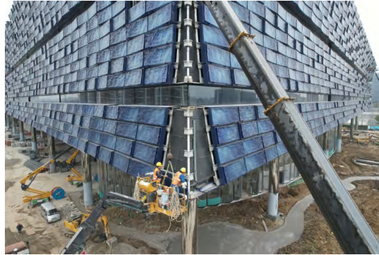
Figure 20 Hoisting of External-Corner Panel Units
