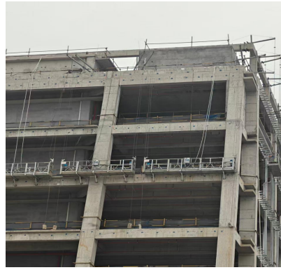
Figure 3 Completed Effect of the Suspended Platform Support Platform
