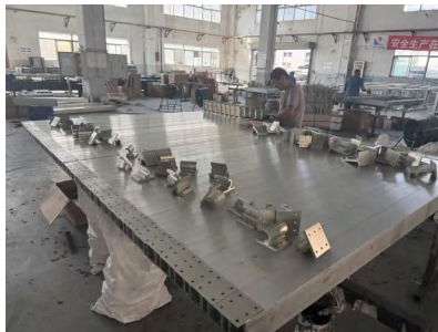
(c) Installation of the Stainless Steel Hanging-Ear Connector
