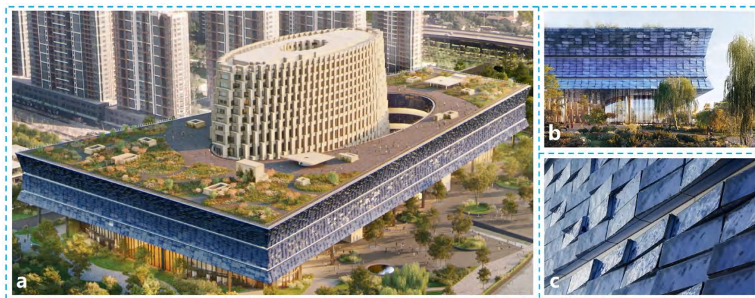
Figure 4 Rendering of the Colored Glaze Curtain Wall of the Architecture (a) Overall Effect; (b) Local Effect; (c) Detailed Effect
