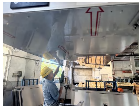
(b) Installation of Backing Plates
